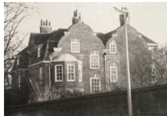
Herschel Lodge before its demolition
